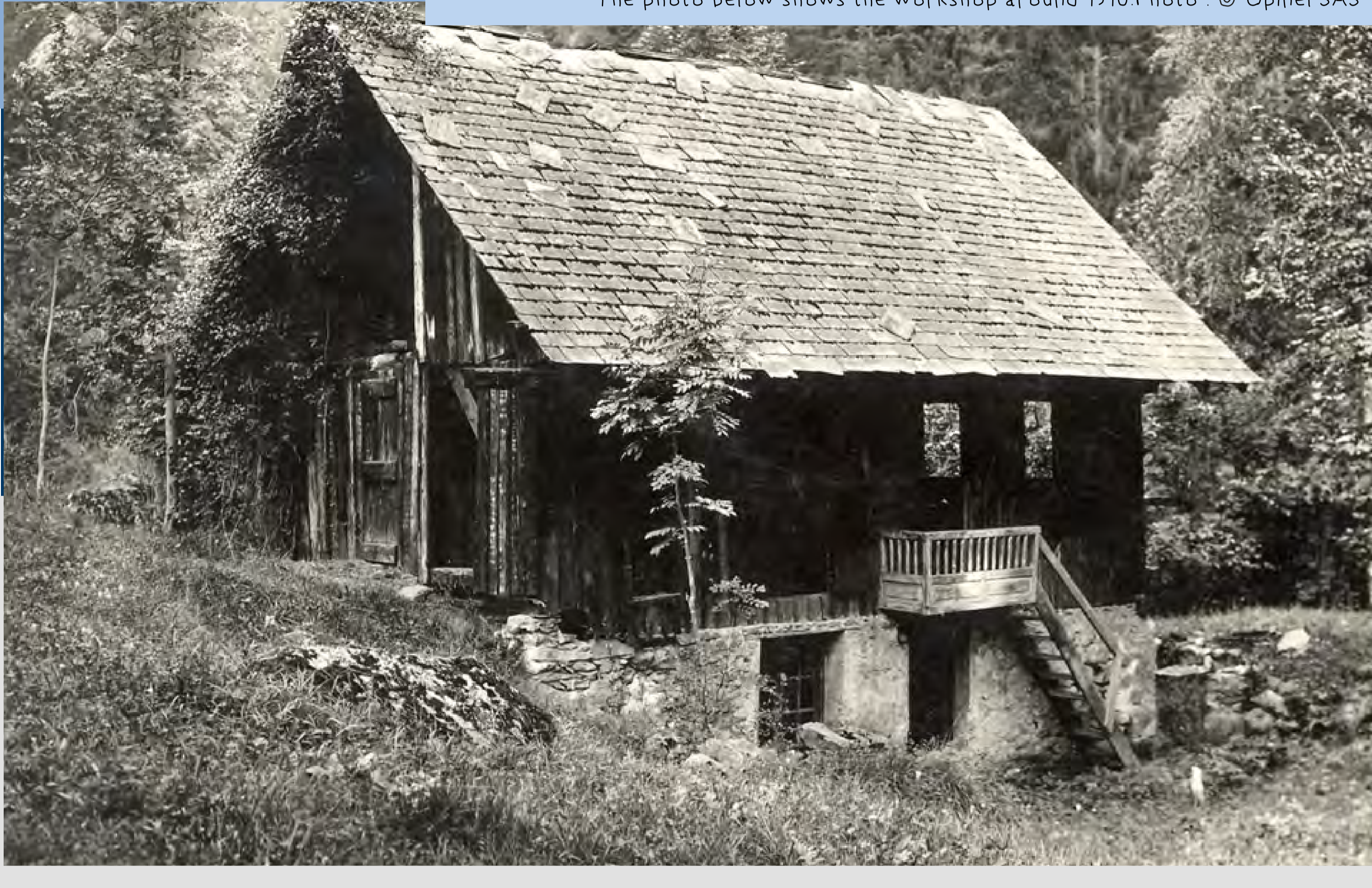
The photo below shows the workshop around 1910. Photo : © Opinel SAS
